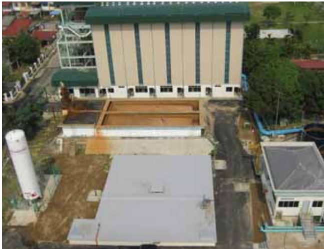
View of water treatment plant in Pintu Geng, Kelantan
