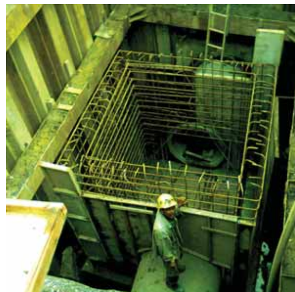
Manhole construction at Kota Kinabalu for the Kota Kinabalu Sewerage Project.
