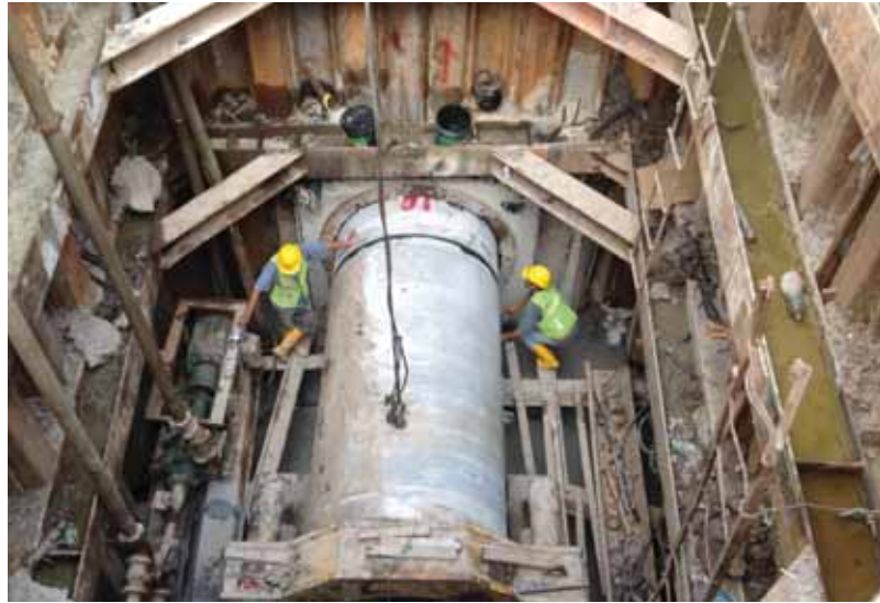
Pipe jacking works for D55 project at Klang, Selangor
