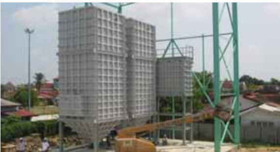
Construction of ozone clarification in Pintu Geng, Kelantan
