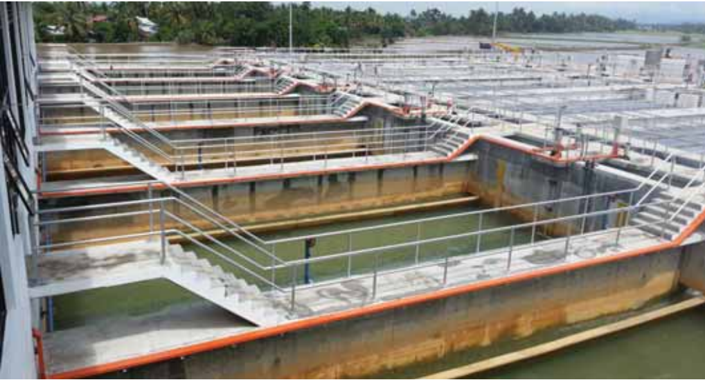
View of 25 MGD Sg. Dua water treatment plant in Pulau Pinang
