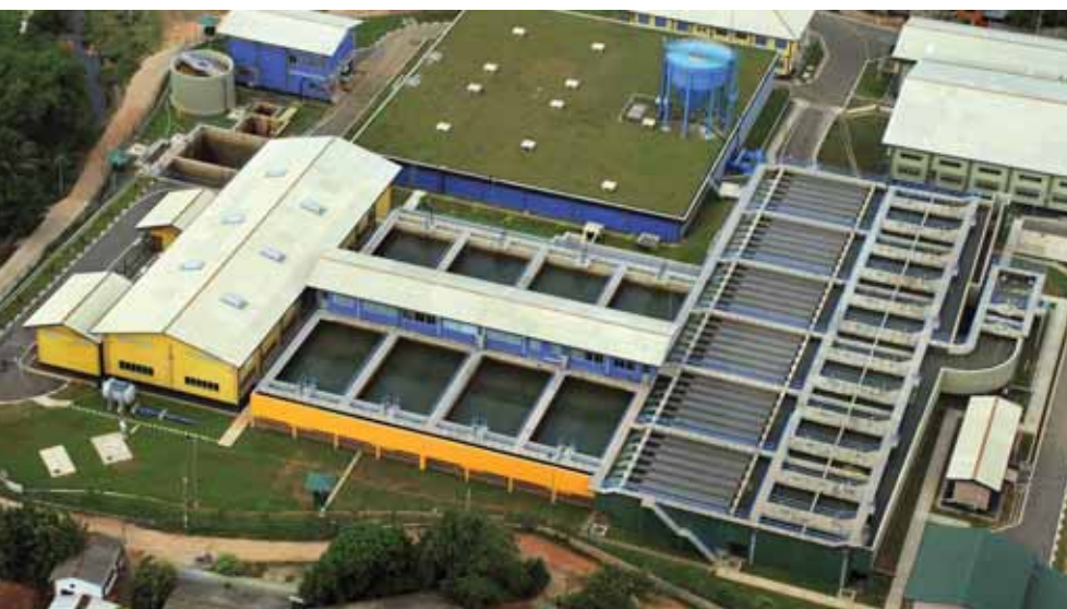
Kelani Right Bank Water treatment plant in Sri Lanka
