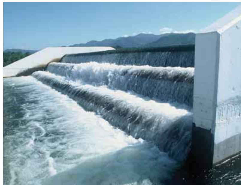
Aerator at Sg. Terip water treatment project
