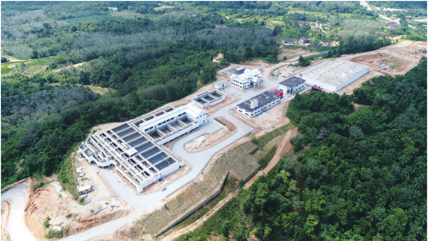
Aerial view of Bukit Berapit Water Treatment Plant of KTU Water Supply Scheme
