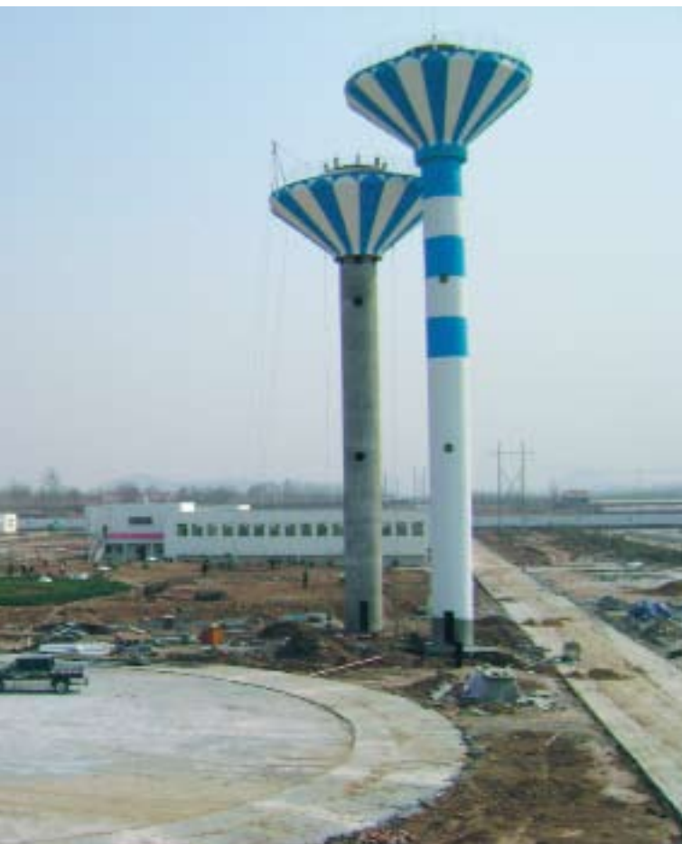
View of Twin Tower water tanks at the new 100 mld Changle Water Treatment Plant, Changle County, Shandong Province, China
