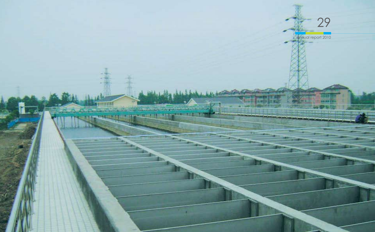
Phase 2 expansion of Haining Water Treatment Plant, Haining City, Zhejiang Province, China with total capacity of 300 mld
