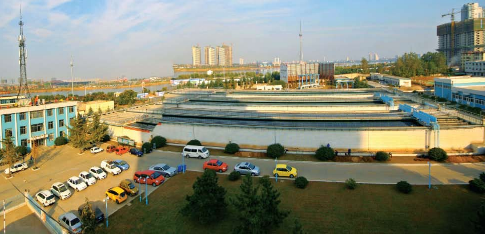
View of 150 mld Linyi Water Treatment Plant, Linyi City, Shandong Province, China
