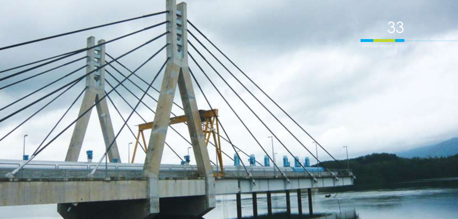
Raw water pumping station on cable stayed deck bridge at Sungai Terip Water Treatment Plant , Negeri Sembilan
