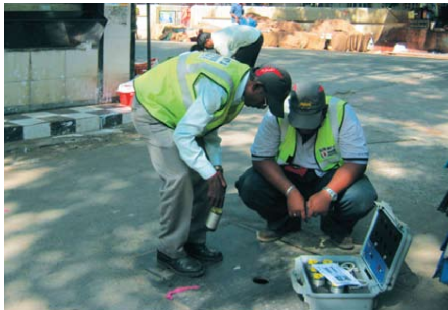
Non-Revenue Water Pilot project in progress in Mumbai, India
