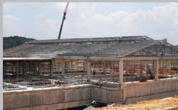
Construction works in progress at Sg. Labu Water Treatment Plant
