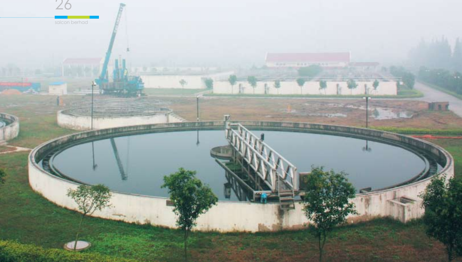
View of Yizheng Rong Xin Wastewater Plant, with capacity of 50 mld in Yizheng City, Jiangsu Province, China
