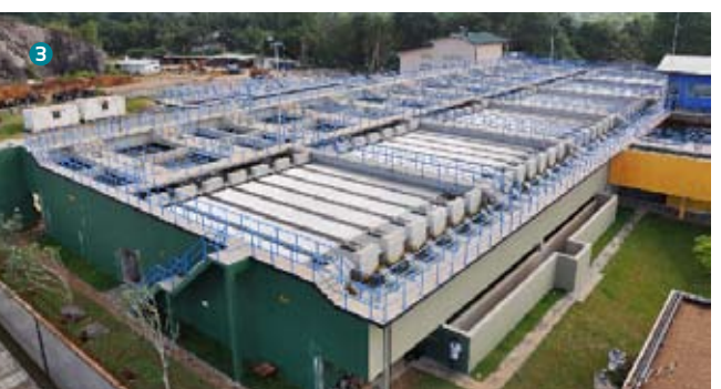
2. Water Treatment Plant at Hambantota, Sri Lanka.
