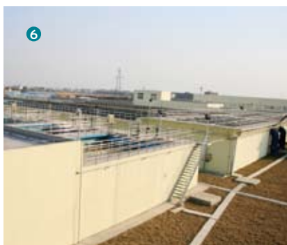
6. View of Qian Yuan Water Treatment Plant, Deqing County, Zhejiang Province, China
