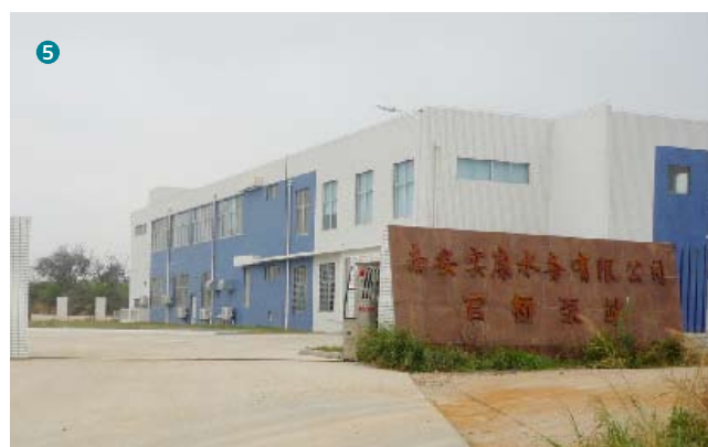
5. Guan Qiao Booster Pumping Station in Nan An City, Fujian Province, China.
