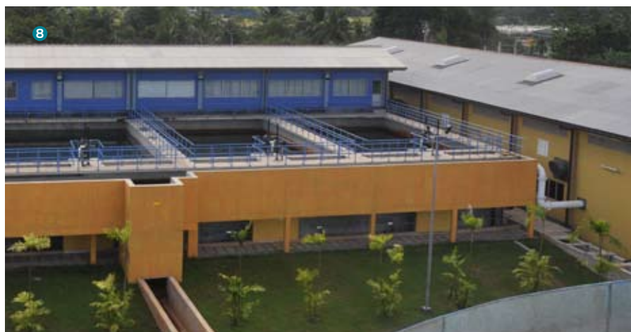
7. View of Wukang Water Treatment Plant, Deqing County, Zhejiang Province, China.
