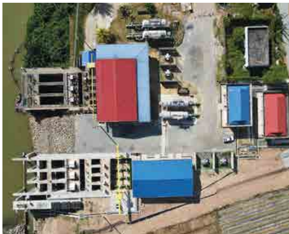
Overview of intake and raw water pumping station at Telibong II WTP
