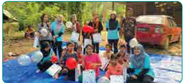
Installation of solar panel for community at Kg. Orang Asli Bukit Tunggul in Lighting Up Our Community Event
