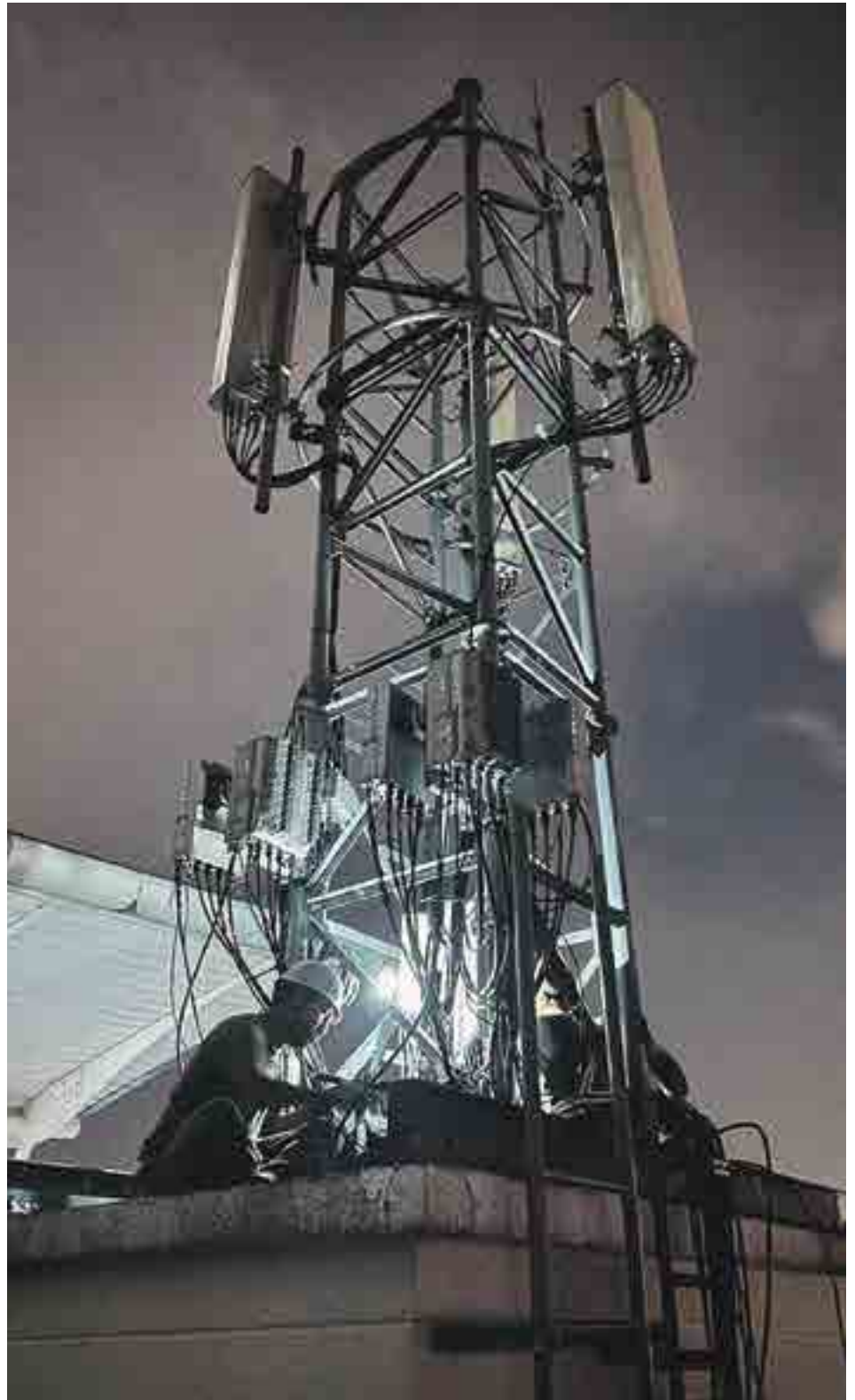
Fiber laying at LRT Taipan
