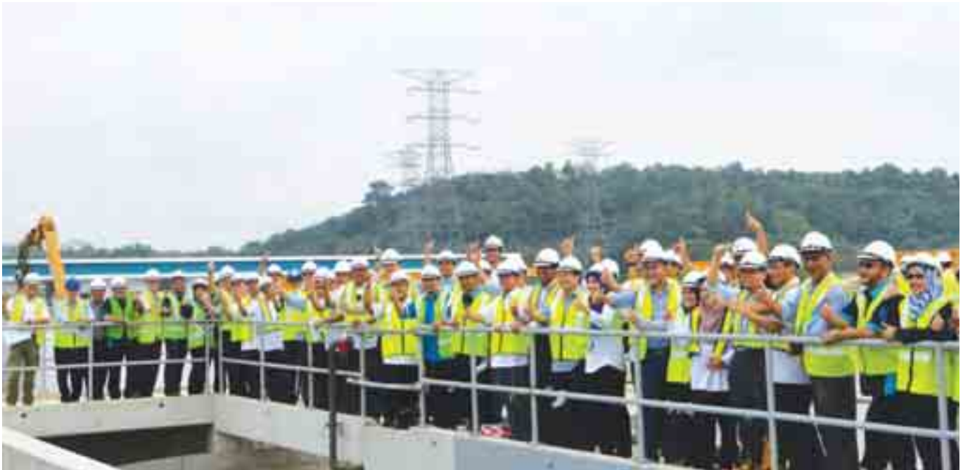
Ministry of Energy, Green Technology & Water team paid a visit to the Langat 2 Water Treatment Plant which is currently under construction
