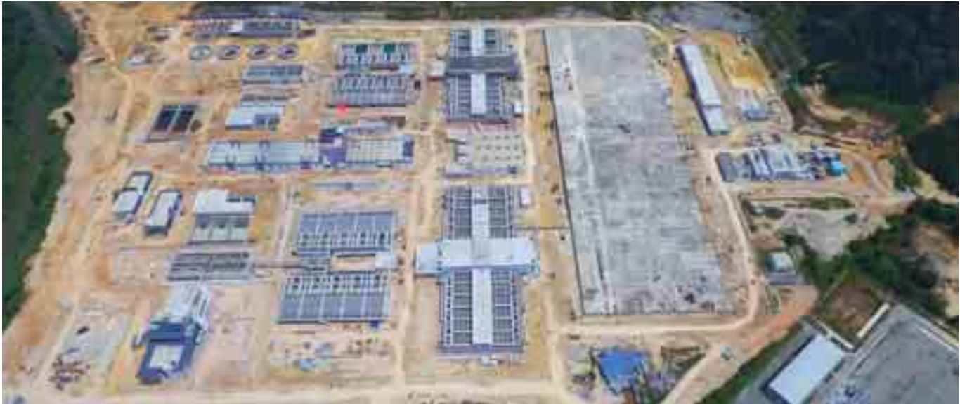
Aerial view of Langkat 2 Water Treatment Plant
