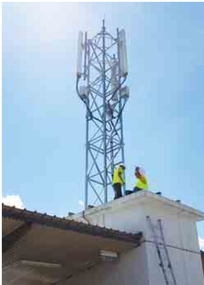
Sectorisation site survey at Gombak LRT station.
