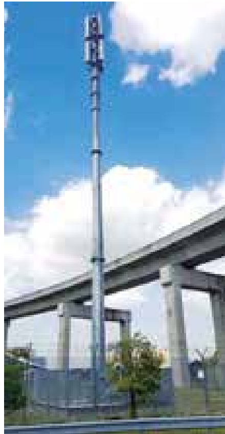
▲ A 30 meter unipole owned by VBT at Lembah Subang LRT Station
