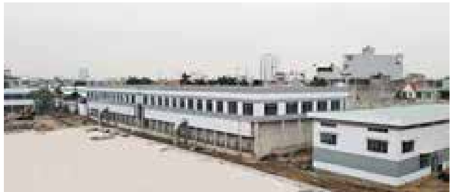
▲ Rehabilitation and upgrading project of Haiphong Water Supply System in Vietnam is expected to be completed in 2020
