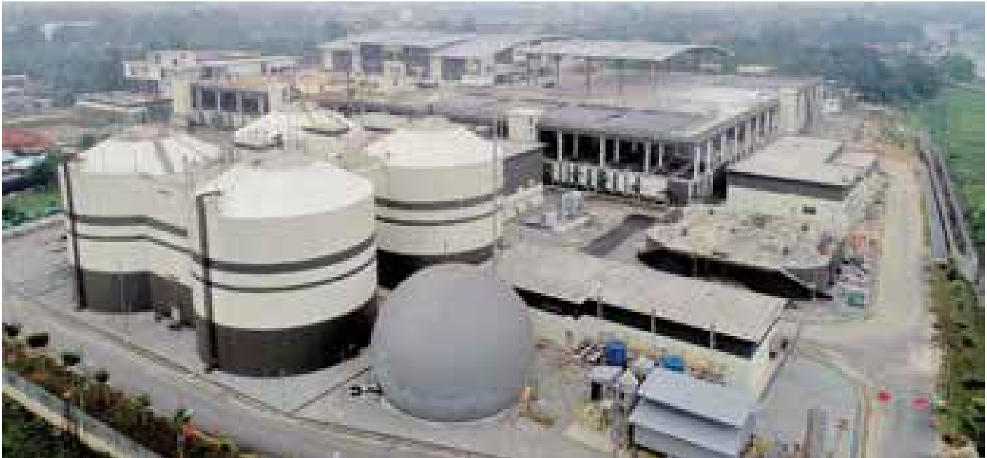
▲ The Langat Centralised Sewage Treatment Plant equipped with Green Technology such as Bio Gas, Solar Energy, Effluent Water Reuse and Rainwater Harvesting
