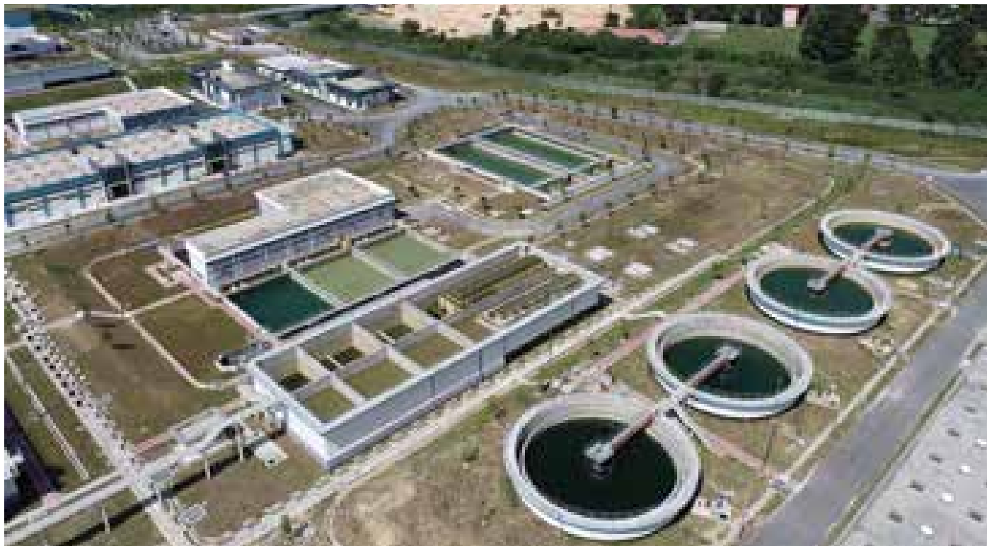
▲ Langkat 2 Water Treatment Plant – the largest single water contract in Malaysia water industry
