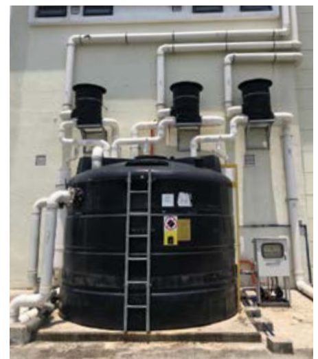
➤ A rain harvesting system with storage capacity of 13,500 litres is used for site washing and plant watering at Langat CSTP
