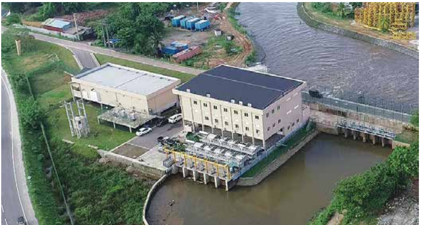
Front view of Ambathale Stormwater Pumping Station in Sri Lanka
