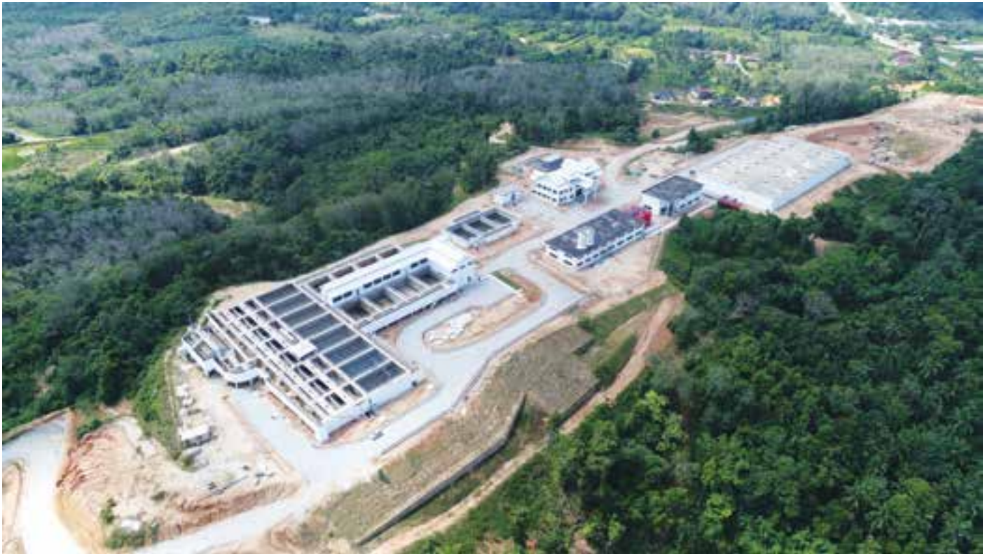
Aerial view of Bukit Berapit Water Treatment Plant of KTU Water Supply Scheme
