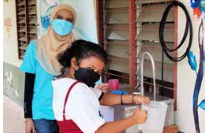
Children of Kg Orang Asli Paya Lebar taking turns to take filtered water from solar-powered water purification system installed by Salcon Berhad
