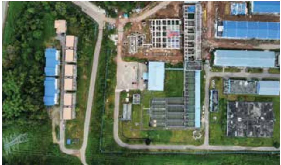
Aerial view of Telibong water treatment plant
