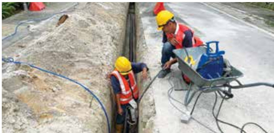
Laying of Vacuum Sewer & Telemetry Cable with total length of 4090m for rehabilitation works of vacuum sewerage system at Bandar Ambang Botanic
