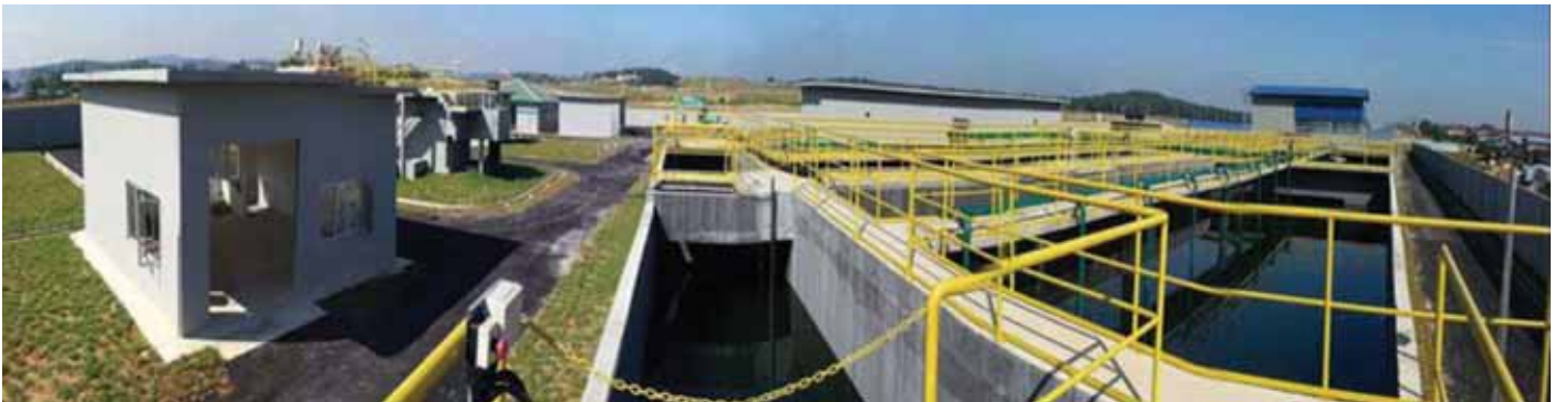
Overall view of Sewage Treatment Plant And Pumping Station At Elmina, Shah Alam, Selangor
