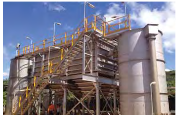
Lamella clarifier system installation in Lao, PDR
