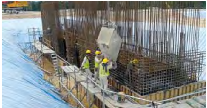
Construction site of Langat 2 Water Treatment Plant project with 1,130 MLD capacity
