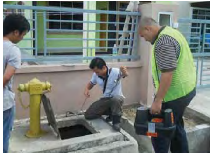
Non-Revenue Water works in Kudat, Sabah
