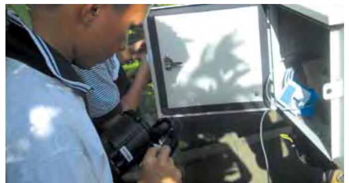
Non-Revenue Water (NRW) works in Kudat, Sandakan
