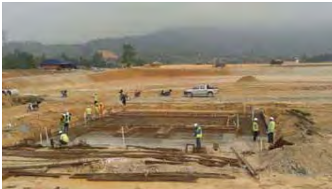
Earthworks at Langat 2 Water Treatment Plant project site
