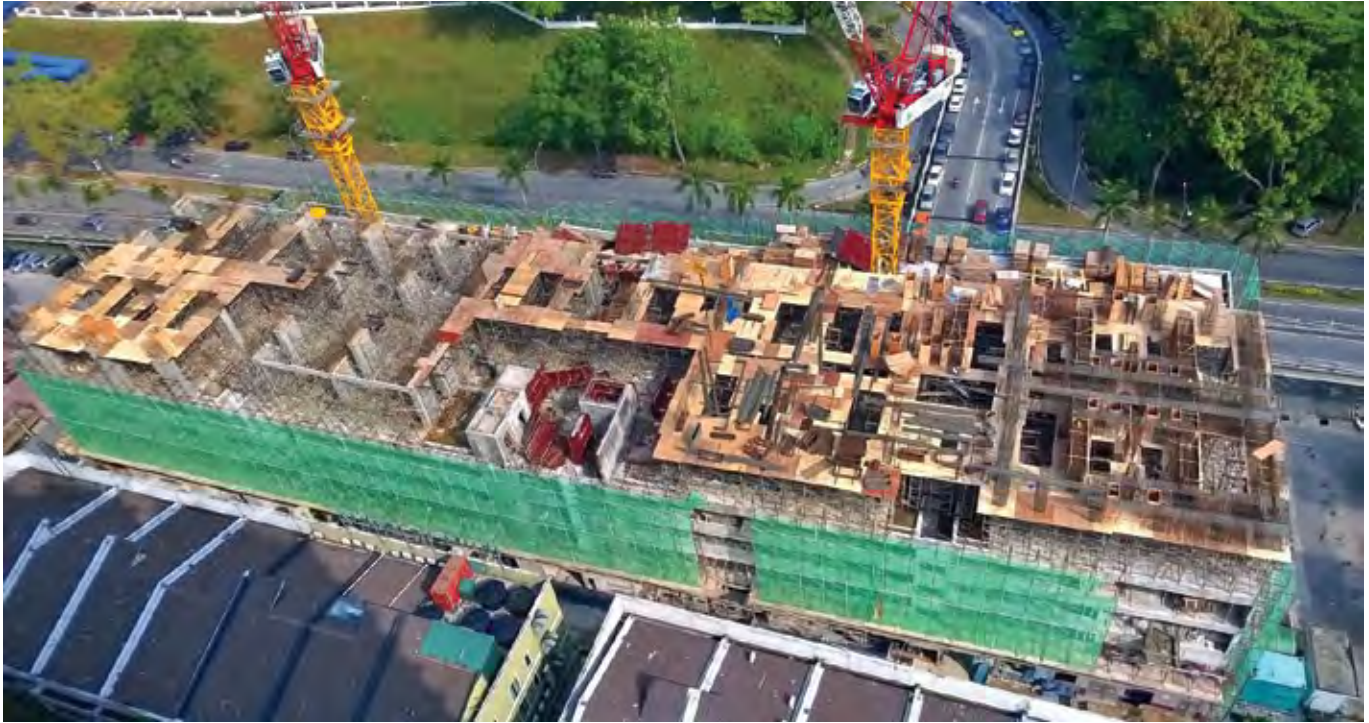
Aerial View of Rés280 construction.
