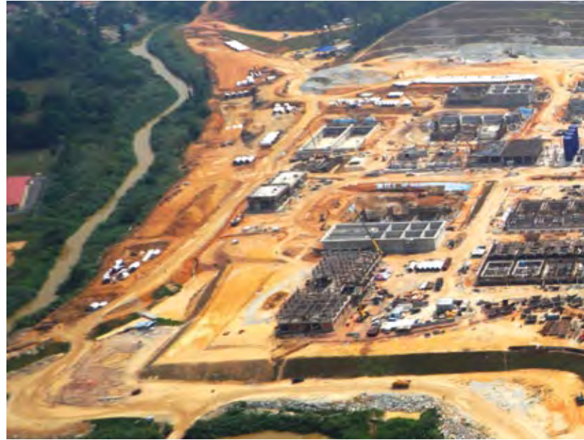
Aerial view of Langat 2 Water Treatment Plant.
