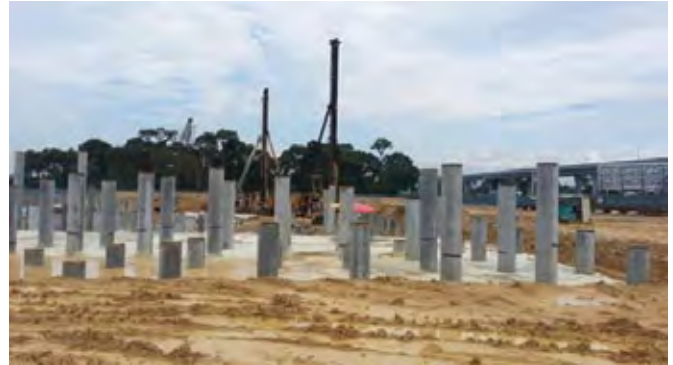
Construction of digester tank piling works at Langat CSTP project site.
