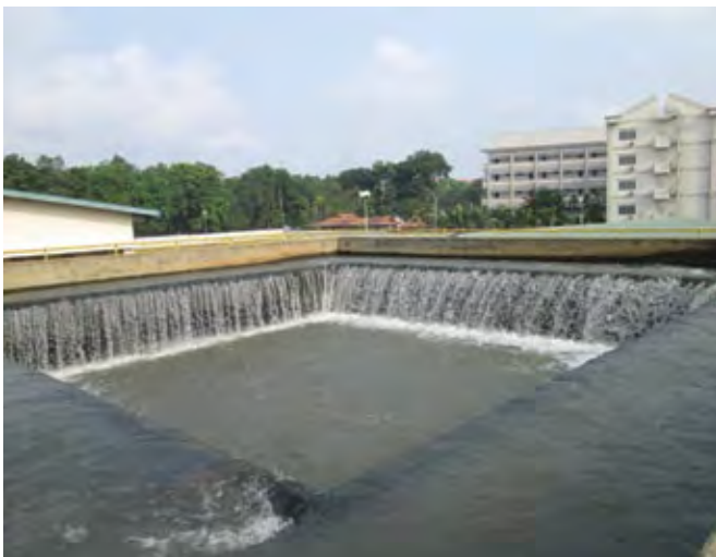
Operation of aerators at Binh An Water Treatment Plant, Vietnam.
