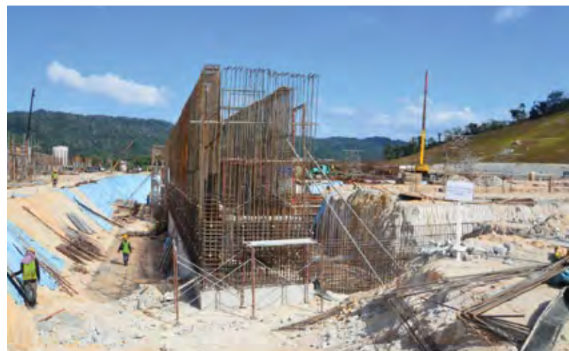
Construction of filter tank at Langat 2 Water Treatment Plant.
