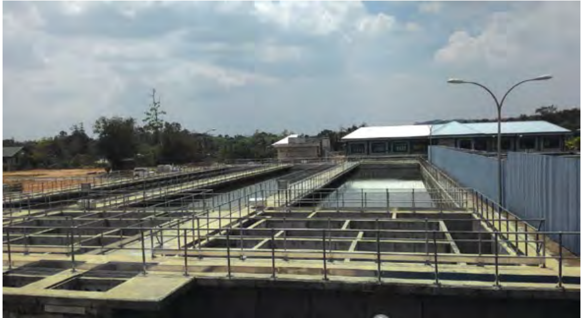
Kalu Ganga Water Supply Project in Sri Lanka was completed in August 2015.
